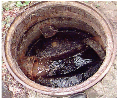
Same 8 inch sewer after cleaning
