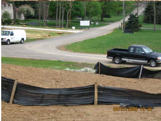
Erosion and Sediment Control at Overlook Quarry
